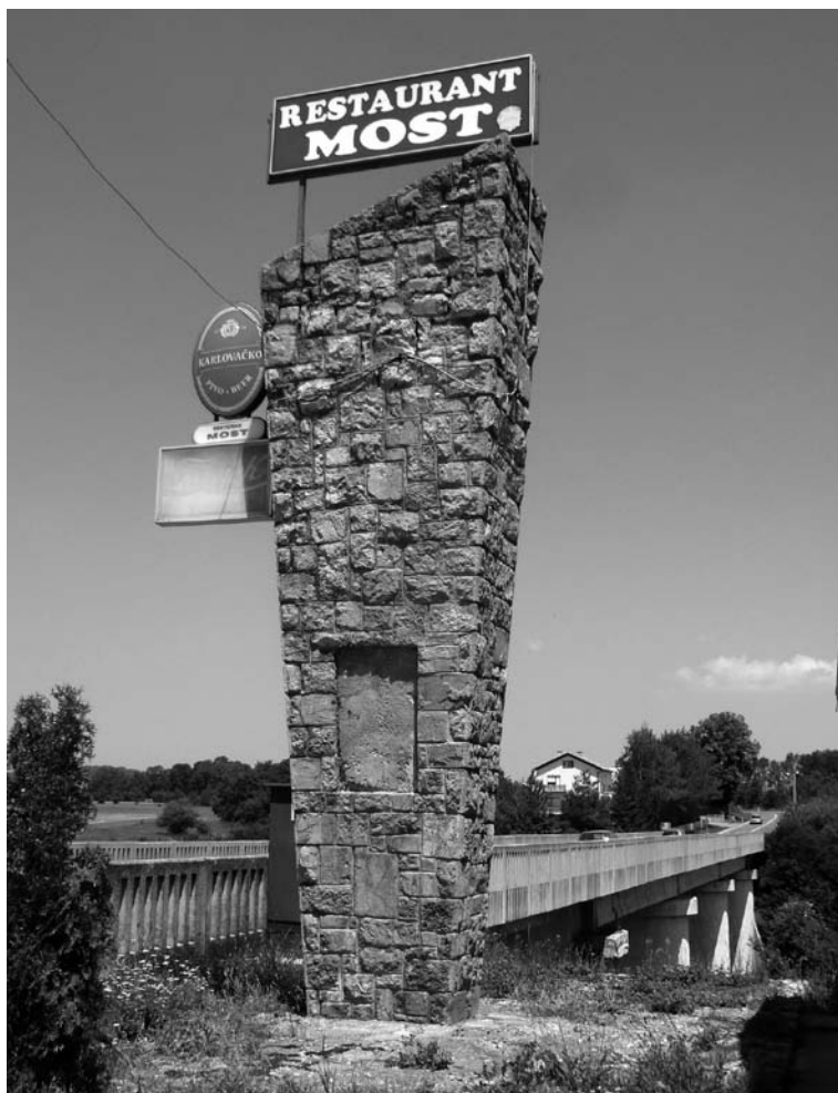
1 Former World War Two monument at the bridge over the River Lika converted into a restaurant sign, photo by Vjeran Pavlaković
