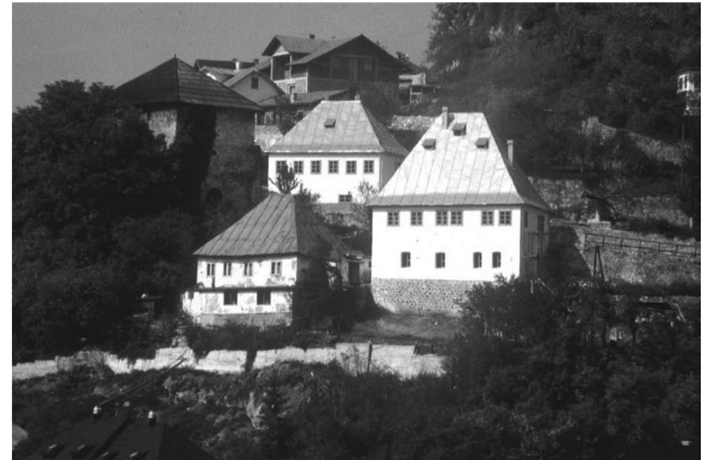
2 Two 18th-century houses in Jajce, Bosnia & Herzegovina, restored 2001-2003
